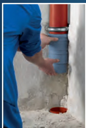
2. Sliding sleeve push over upper tube
