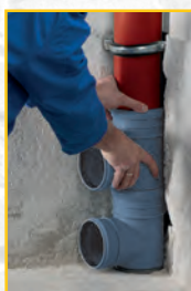
4. Push the sliding branch into the sleeve of the plug-in branch
