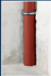
1. Existing pipe 33 cm cut out
