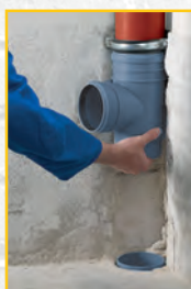
2. Sliding sleeve push over upper tube
