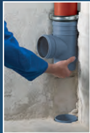
2. Sliding sleeve push over upper tube
