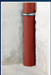
1. Existing pipe 33 cm cut out
