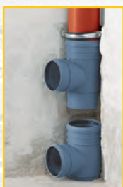
3. Plug the plug-in branch into the lower tube
