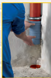
2. Sliding sleeve push over upper tube
