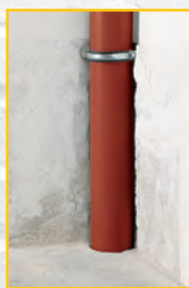
1. Existing pipe 33 cm cut out
