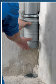
2. Sliding sleeve push over upper tube
