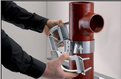
1. Both clamp halves must close the pipe ends evenly
