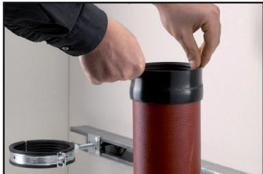
1. Put the sleeve on the end of the pipe. The middle spacer ring of the seal rests on the pipe.
