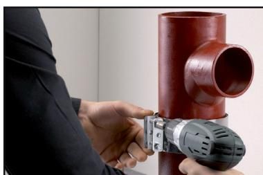
6. Place the connector and tighten it evenly on both sides using a screwdriver.
