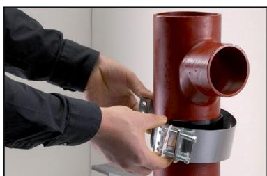
5. Attach the metal band and fix it with screws.
