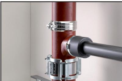
3. Mark the connection pipe to the required installation depth, apply lubricant and push it in.
